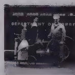
An acetylene torch won't burn through its twenty-gauge sides.
