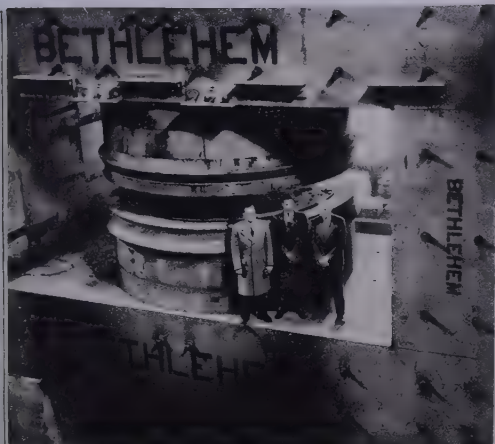
Prof. E. T. Booth (left), executive director Columbia's nuclear physics research center, stands with two other engineers on the partly finished 2,500-ton, 400-million-volt cyclotron for atom research.
